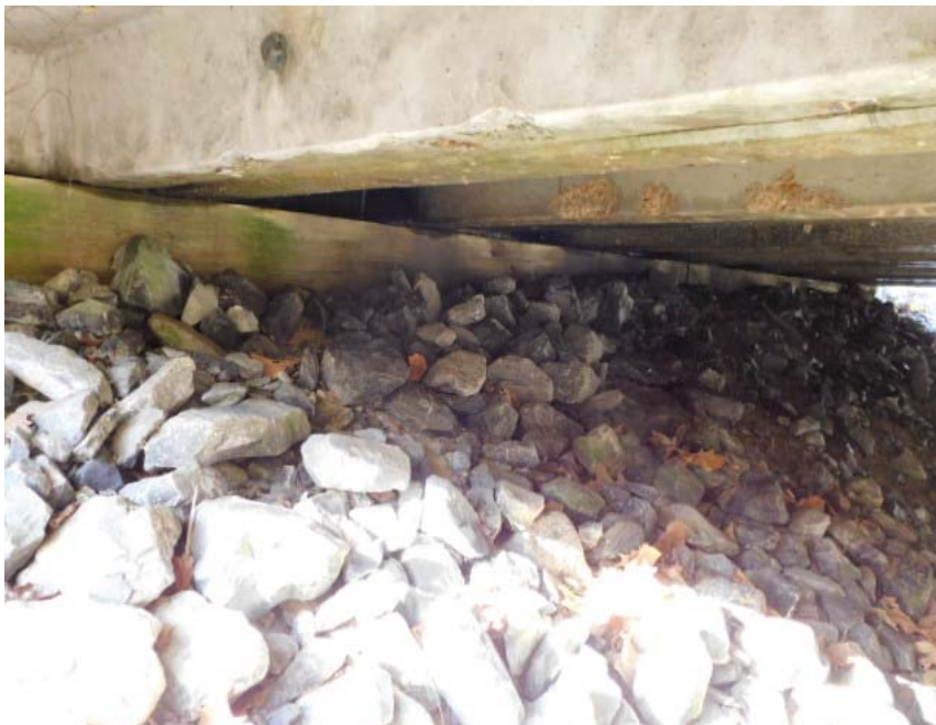
LEFT SIDE END OF CAP ABUTMENT # 1 DECAYED
