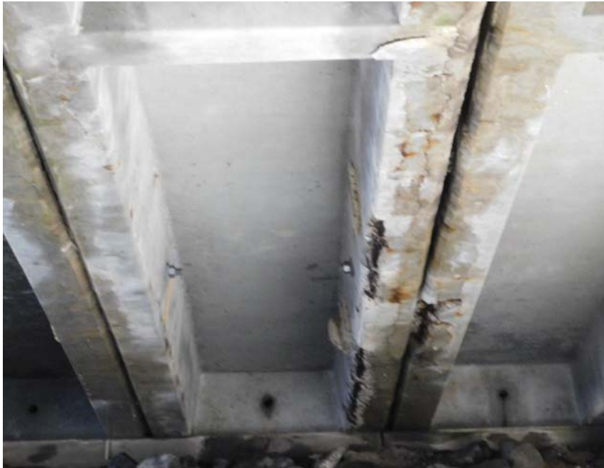
SLAB "D" SPAN # 2 SPALLED TO STEEL
