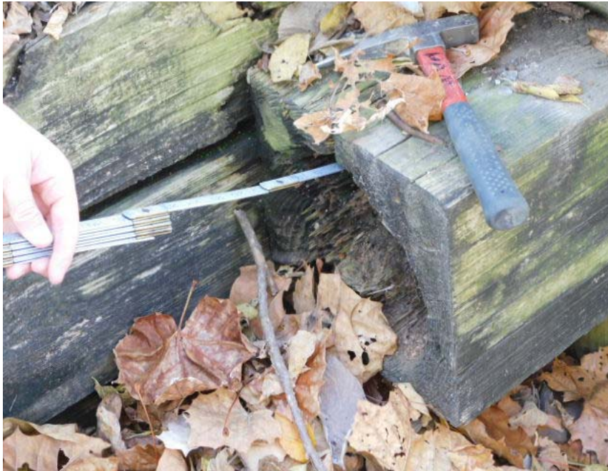
LEFT SIDE END OF CAP ABUTMENT # 1 DECAYED
