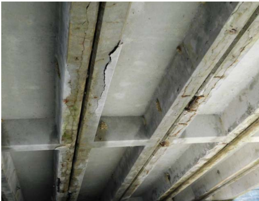
SLAB "D" SPAN # 2 SPALLED TO STEEL
